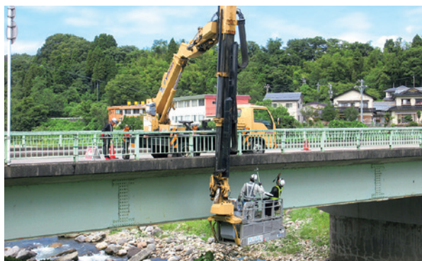
橋梁の近接目視点検
