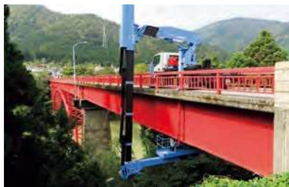
橋梁の近接目視点検
