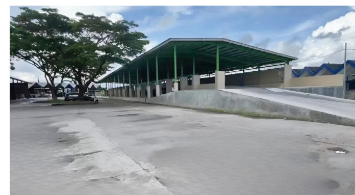
The compost plant is 100 meters long and can process up to 50 tons of food waste per day, producing 17 tons of compost.
